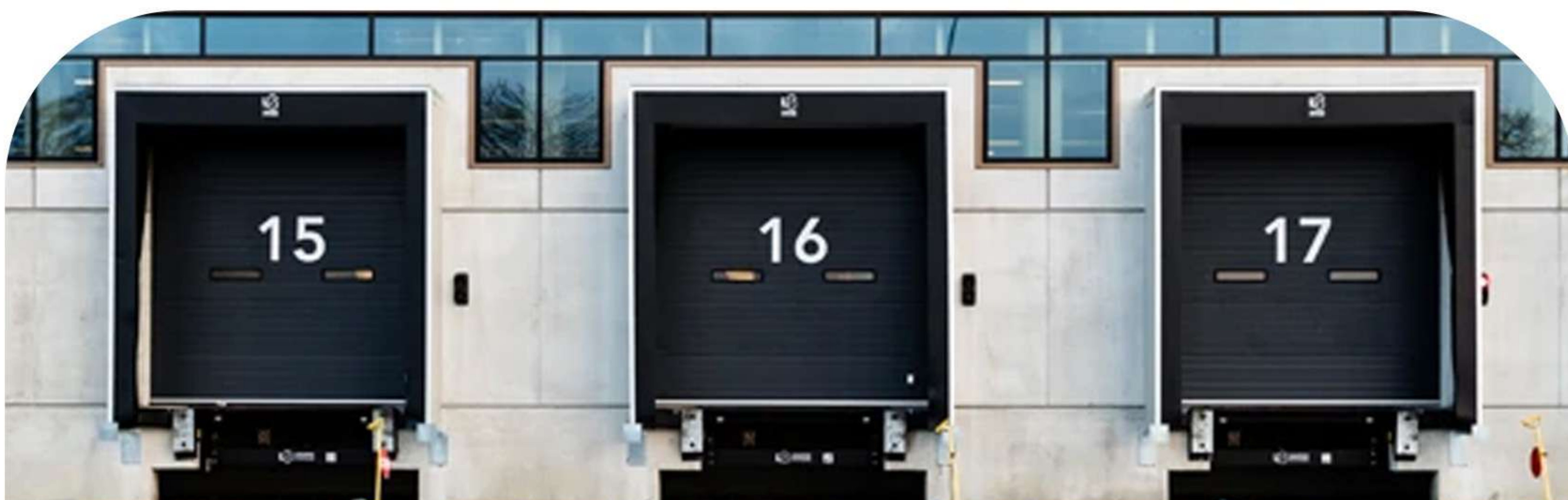
DOCKING BAY & WAREHOUSE SOLUTION
